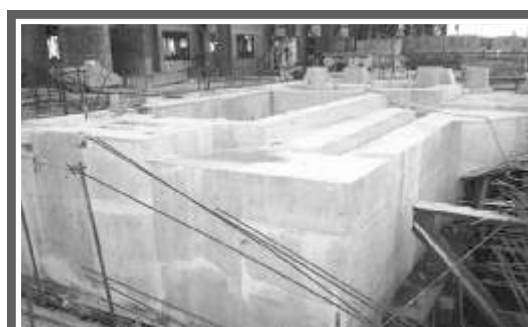
TG foundation for Captive Power Plant of Bhushan Energy Ltd., Meramandali
