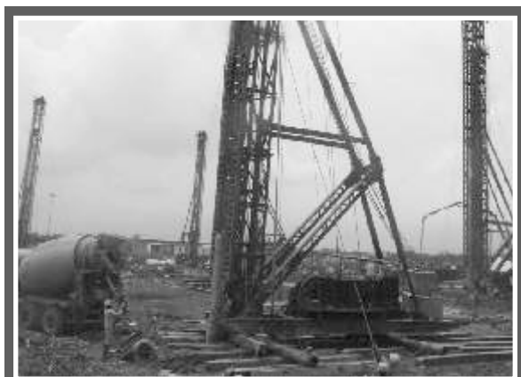
Power Plant of Haldia Energy Ltd.
