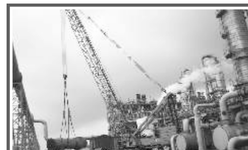
Equipment Erection at MCC PTA, Haldia Project
