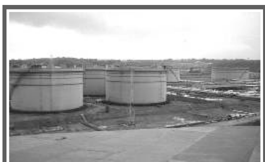
Tankage Work at MRPL, Mangalore
