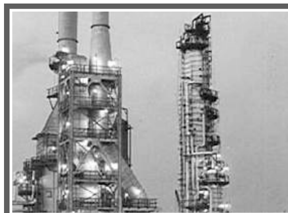
VDU Furnace at IOCL, Haldia
